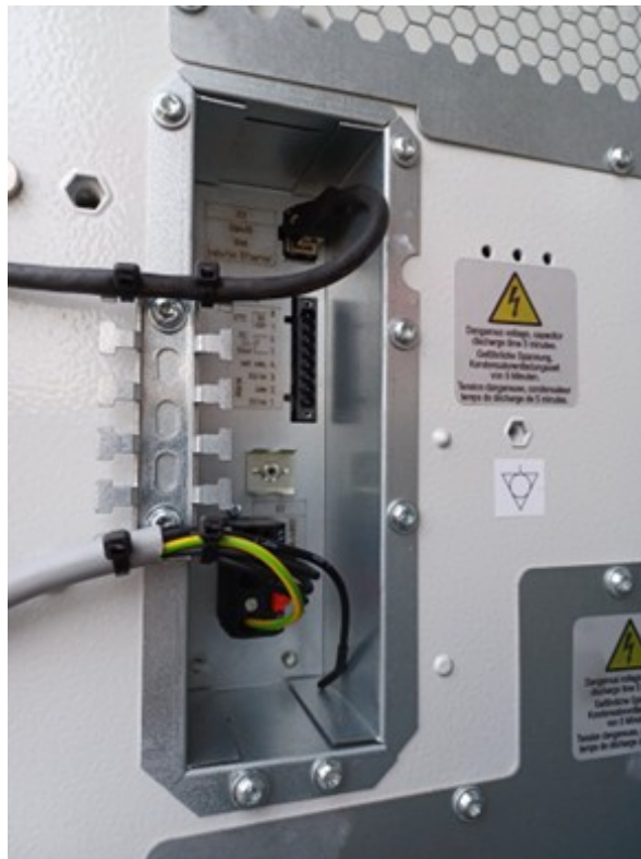
Image 42. Connecting the room air conditioning
